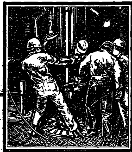
Drillers at work on the first oil operated Beatrice A Platform.
